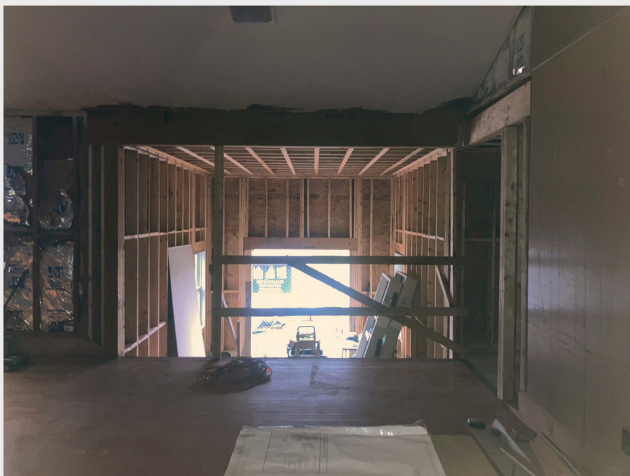
A look at the framing of the new accessible entrance
